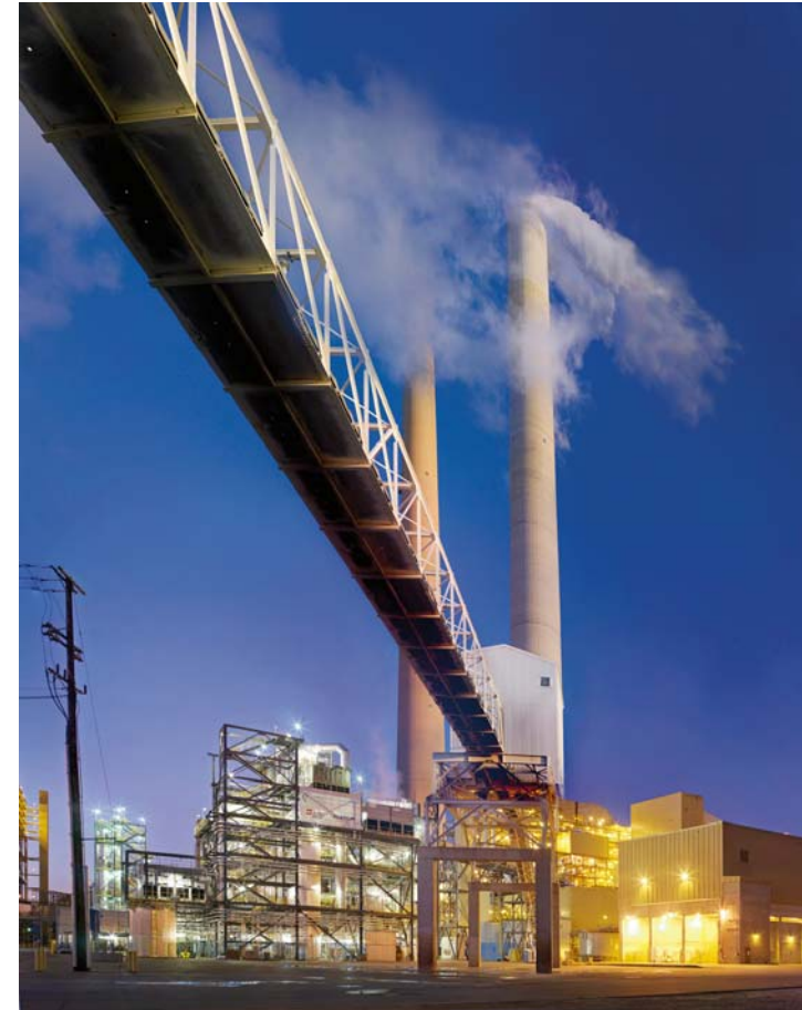
Carbon Capture and Storage project Mountaineer Plant - New Haven, WV
