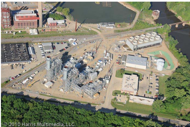
J. Lamar Stall Combined-Cycle Gas Plant
