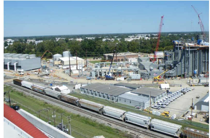
J. Lamar Stall Combined-Cycle Gas Plant
