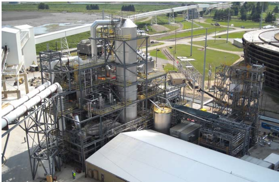
Carbon Capture and Storage Project – Mountaineer Plant (WV)
