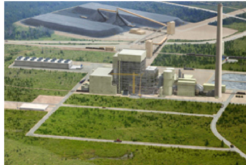
A rendering of the John W. Turk, Jr. ultra-supercritical coal power plant now under construction in Arkansas
