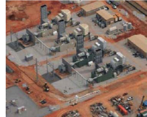
Harry D. Mattison Plant - commercial operations achieved in 2007
