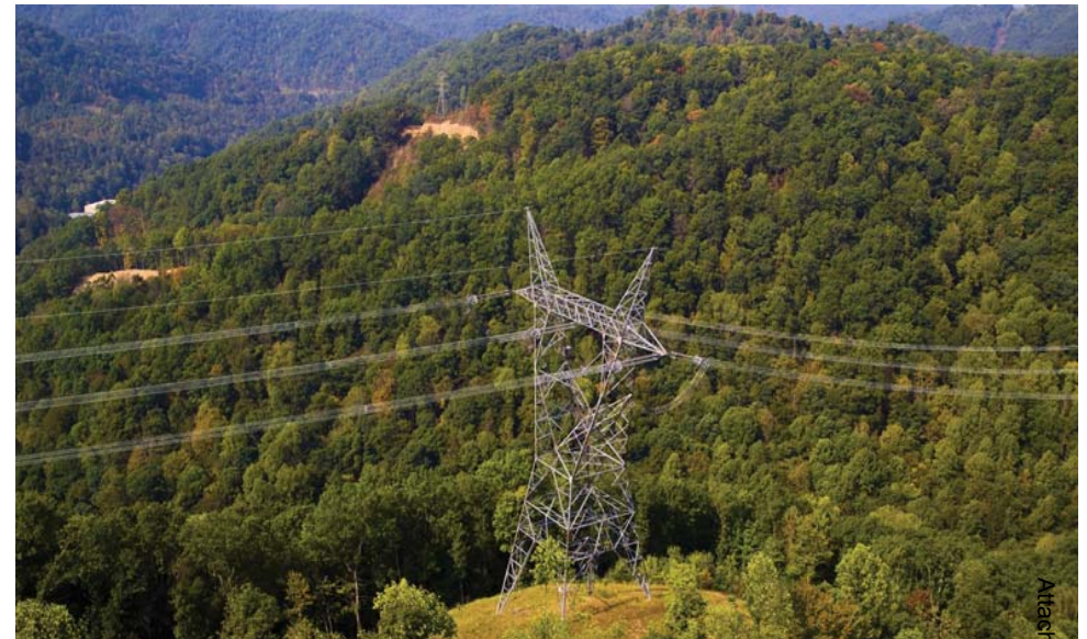
765-kV Transmission Line – Wyoming-Jacksons Ferry (WV)
