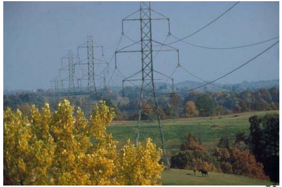
345-kV Transmission Line
