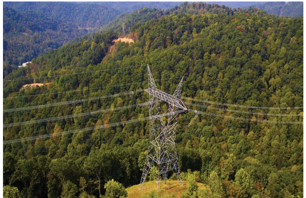
765-kV Transmission Line - Wyoming-Jacksons Ferry (WV)
