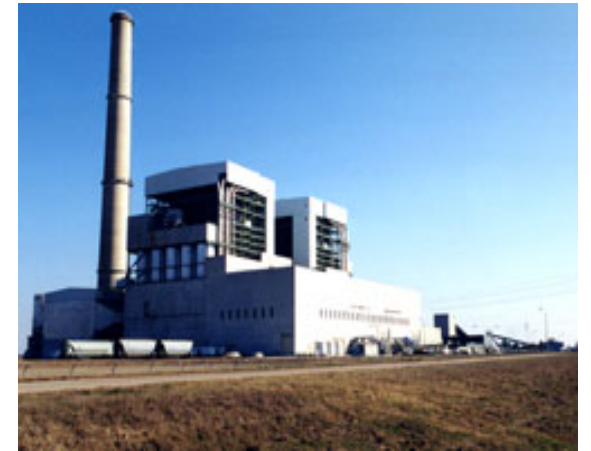
Northeastern Plant - Oologah, OK
