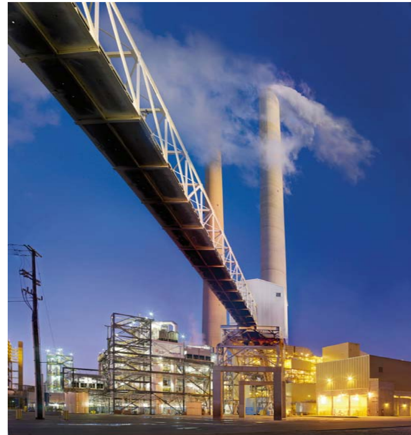
Carbon Capture and Storage project Mountaineer Plant - New Haven, WV
