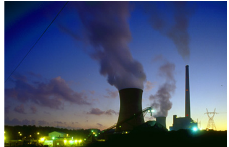
Big Sandy Plant
