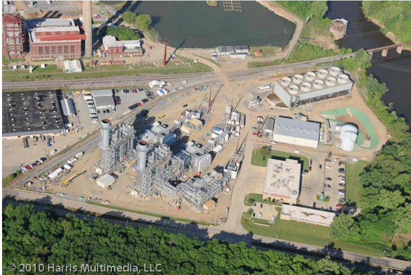
J. Lamar Stall Combined-Cycle Gas Plant
