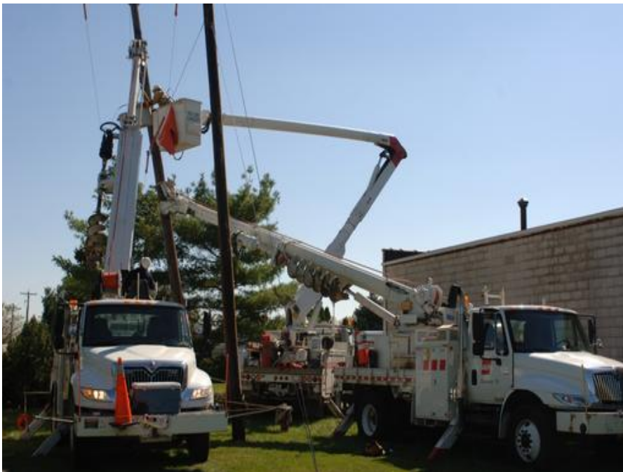
Hurricane Ike Restoration
