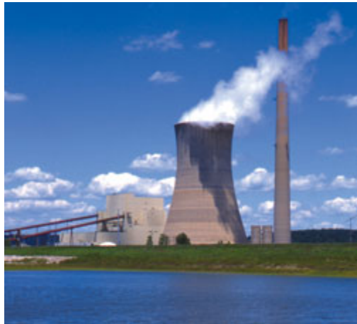
Mountaineer Plant - New Haven, WV
