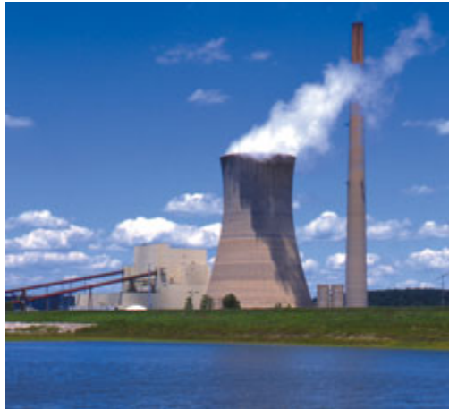
Mountaineer Plant - New Haven, WV
