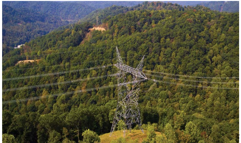
765-kV Transmission Line – Wyoming-Jacksons Ferry (WV)
