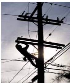
One of the largest U.S. electricity distributors
