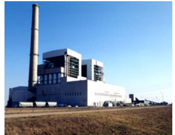
Northeastern Plant - Oologah, OK
