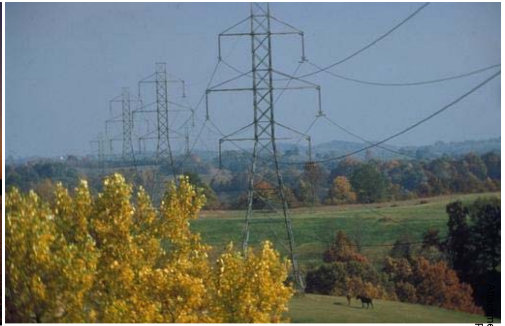
345-kV Transmission Line
