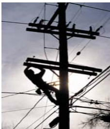
One of the largest U.S. electricity distributors
