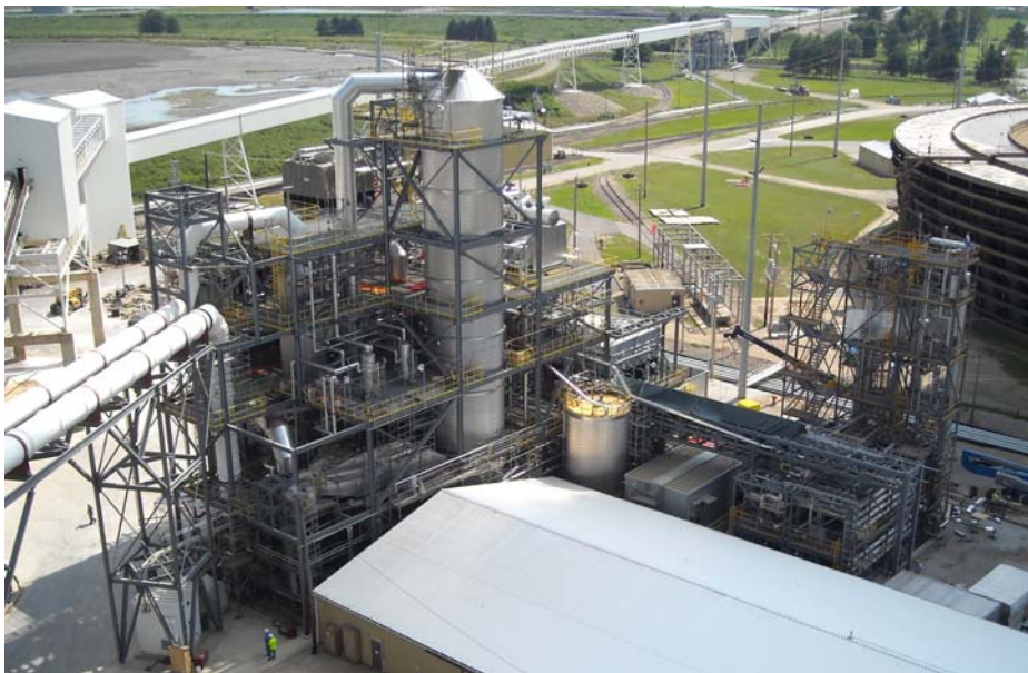
Carbon Capture and Storage Project – Mountaineer Plant (WV)
