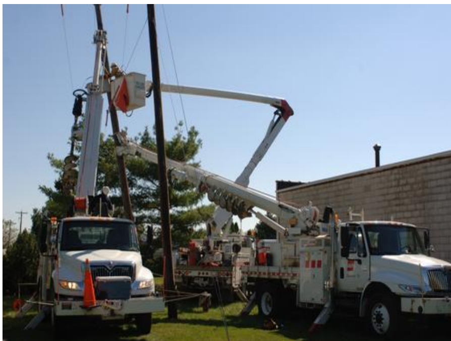
Hurricane Ike Restoration
